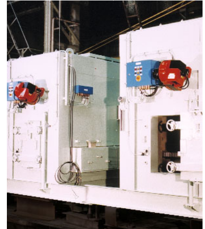
Waste incinerator with two L1 burners onboard the luxury liner MS Empress
